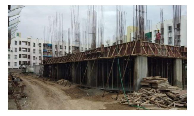
In Block C1: Sixth Floor level slab shuttering work on progress.
