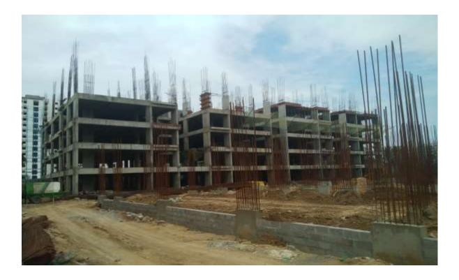
In Block D3: Second floor Level Slab Concrete 100% Completed. Third Floor level Slab First Half Completed.
