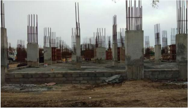
In Block A2: Pile Cap & Plinth beam Work Completed and Earthwork Backfilling on progress.
