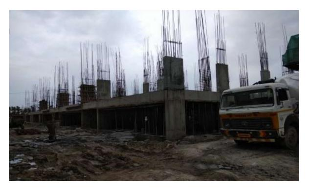
In Block D1: Pile Cap Works Complete. Short Column work and Earthwork backfilling for on Progress.
