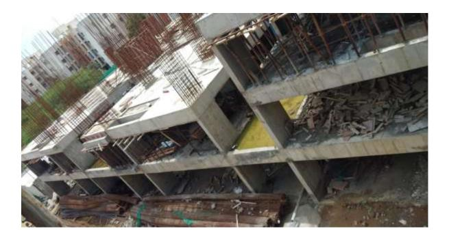
In Community Hall: Pile cap Concrete casting completed. Stilt floor Column work on progress.
