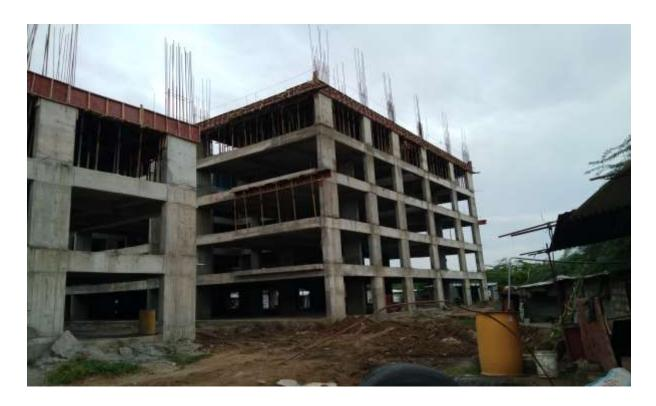
In Block C2: Third Floor level First Half Concrete Complete & Second Half Shuttering complete. Shuttering & Bar bending work on progress for First Half of Fourth Floor level slab.
